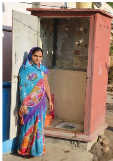
Image 19. Pre-fabricated toilets with twin pits. (Credit: SSP)
