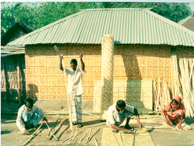
"Houses that incorporate corrugated sheets, like this one in Bangladesh, are more resistant to natural disasters."
